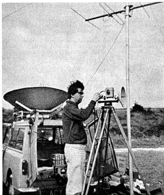
The date: 5 September, 1969. The place: the white cliffs of Dover. The person: Dr Dain Evans, G3RPE. And the occasion? The cross-Channel QSO on 3cm between G3RPE/P and F2FO/P. Contrast the size of the 3cm "signal squirter" with the 2m talk link aerial above. (Full story: page 792, November)
